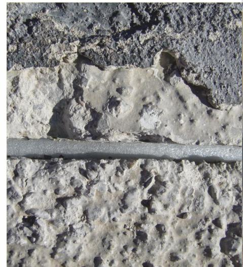
High performance special sealants are used in door and window corners, precast structures and the connection edges of two different materials in buildings.
